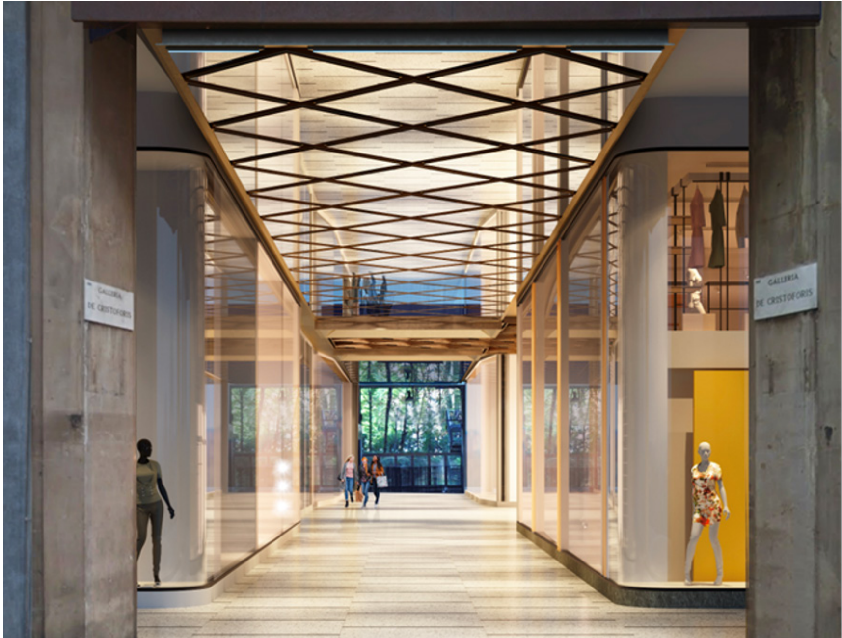
RENOVATION PROJECT OF THE GALLERY
